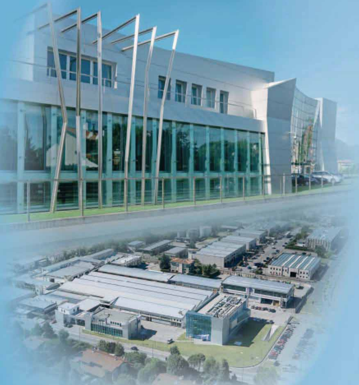
LOVATO Electric headquarters in Bergamo, Northern Italy
